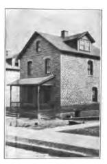
FIG. 72.—STEEL TOWN IN PENNSYLVANIA. SUB-STANTIAL HOLLOW TILE AND BRICK HOUSE.
